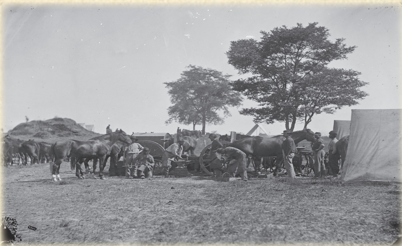
This vehicle is called a battery forge. This vehicle helped to keep iron parts in working condition.
